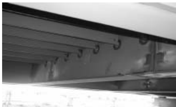
Fig. 3 Ballasted railway deck
