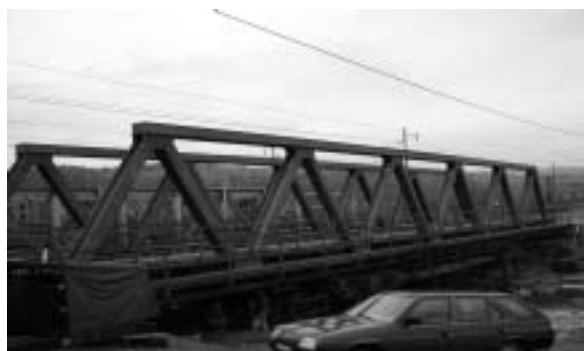
Fig. 4 Truss bridge structure for medium span
