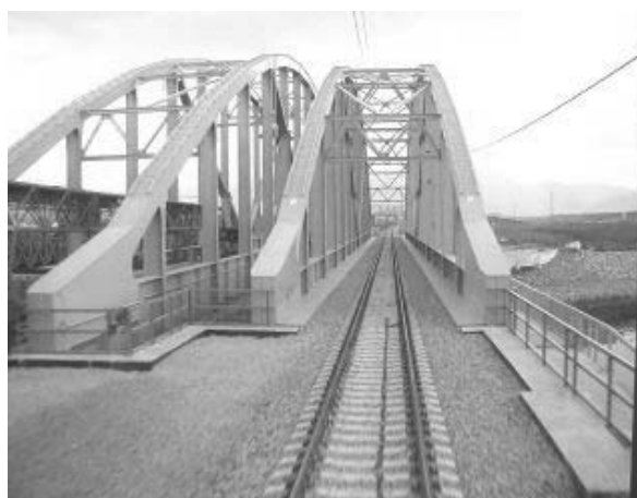
Fig. 5 Bowstring arch system for larger span
